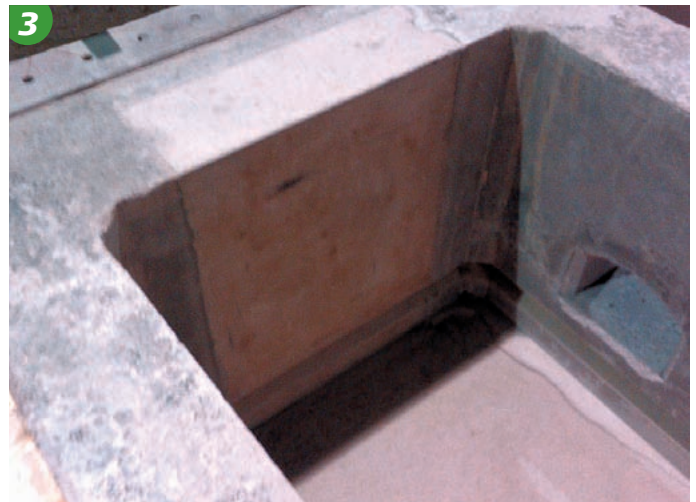
Fig. 3 • Precast big block sidewall melter
